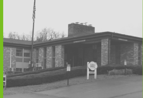
BRIDGES™ and Prevention Building
