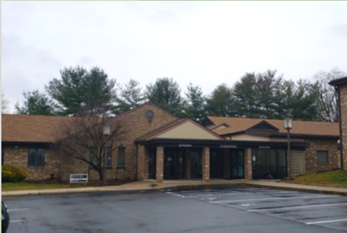
Administration and Permanency Building
