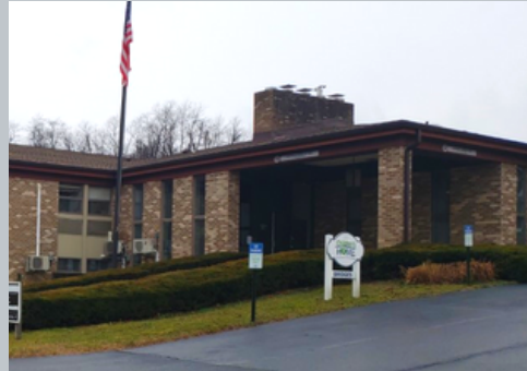
BRIDGES™ and Prevention Building
